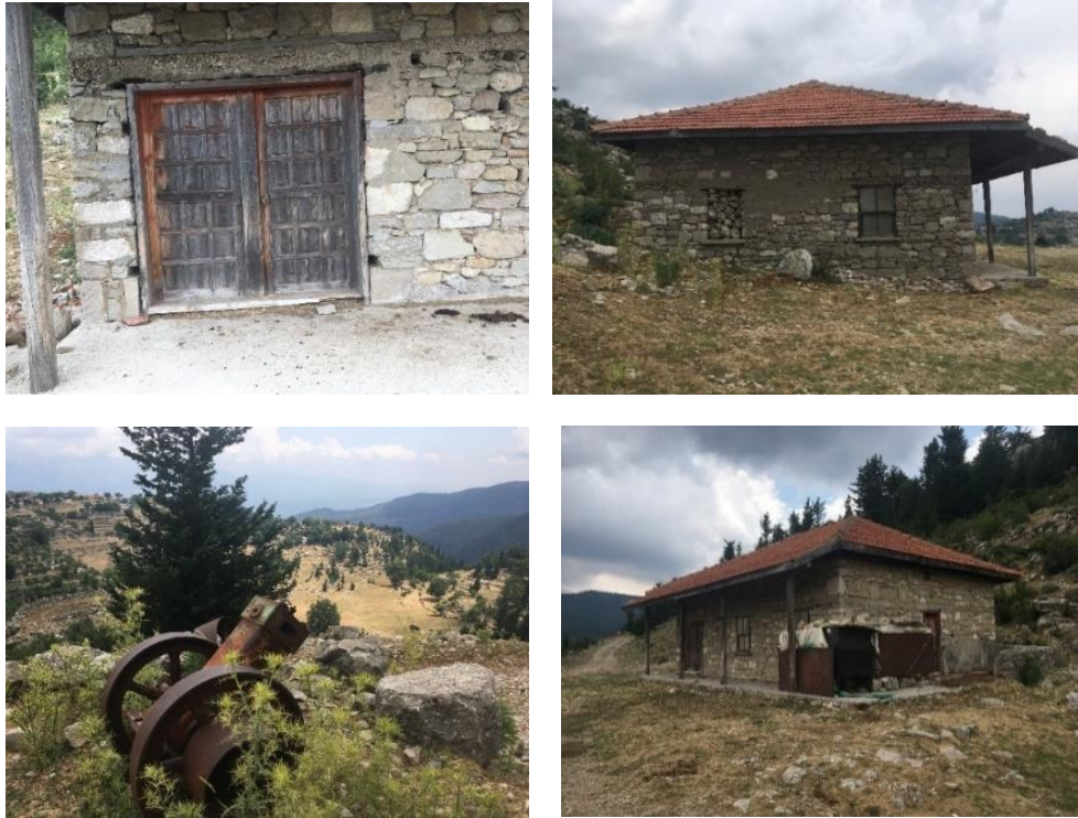
Figure 3.58: The mill that was constructed with cooperative, author, 2021.
