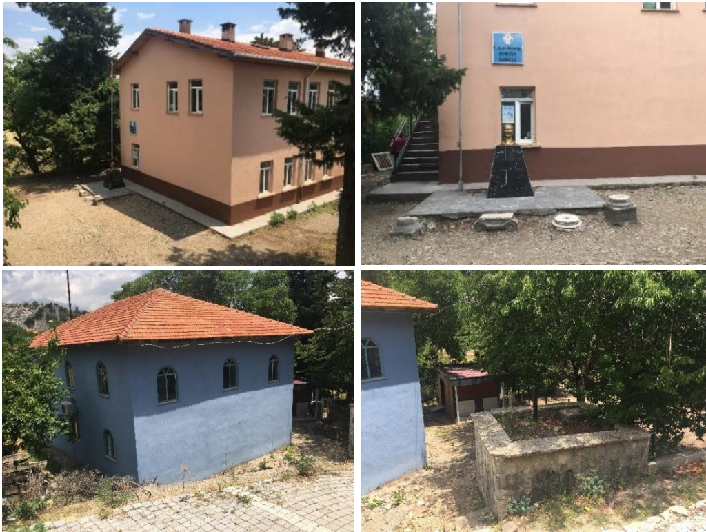
Figure 3.59: The school and the mosque with well, author 2021.
