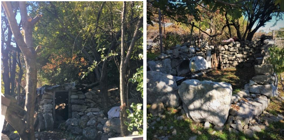
Figure 3.78: Carpenter shops in ruins, author, 2021.
