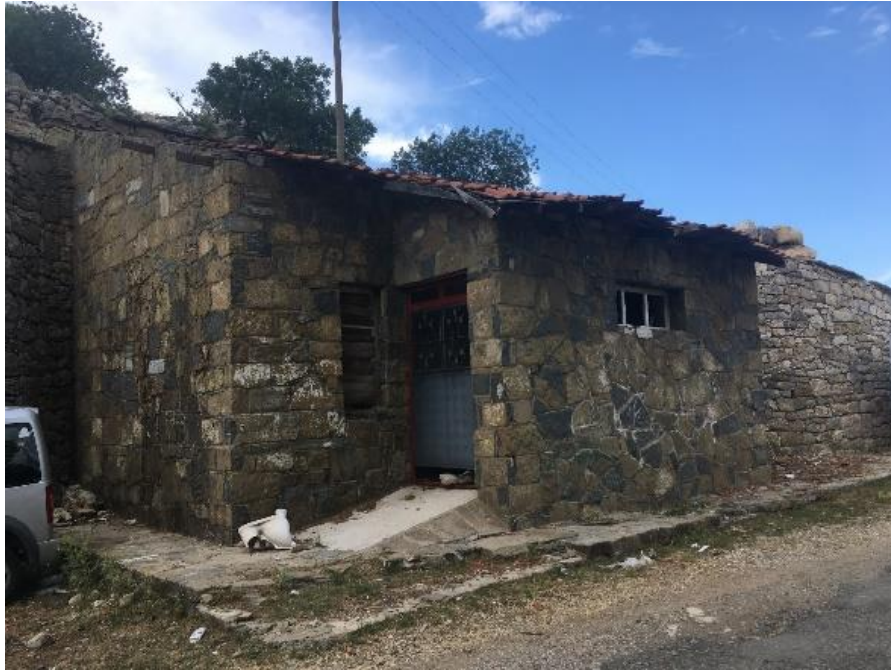
Figure 3.83: Public toilet unit that is not used now, author, 2021.
