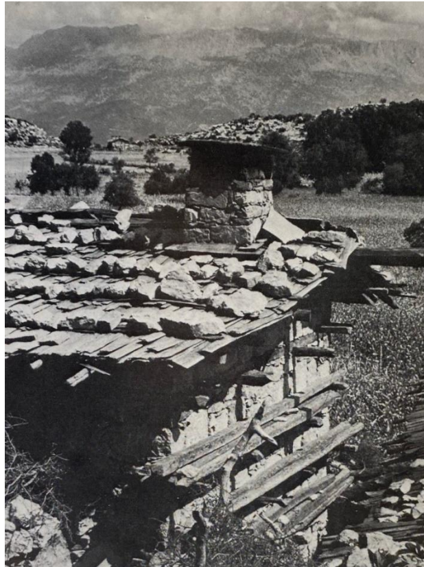
Figure 3.43: The stones on the roof (Machatschek, Schwarz, & Dörner, 1981).
